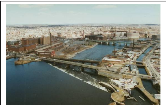
View of Lawrence above the Great Stone Dam looking east.
